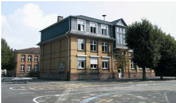
administration buildings, schools, prisons, hospitals, roads etc.
